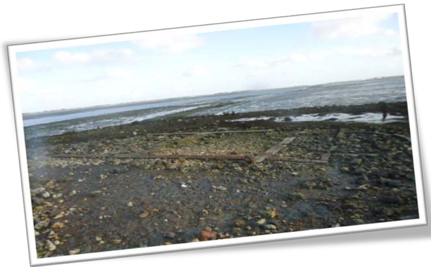
"This is all that's left of the old oyster house. You can see the foundations to the old house"
